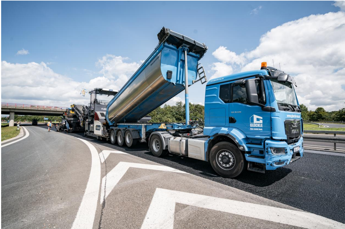
Figure 2: Asphalt works on B286 near Schweinfurt
