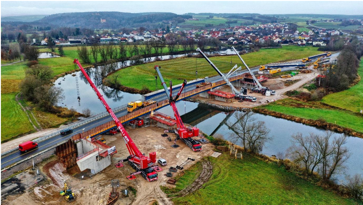
Figure 1: Bridge construction on major interurban road near Regensburg
